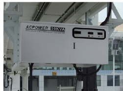
Airport Apron / Hangar
